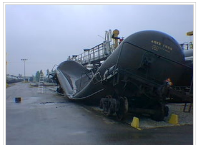
Collapse of railroad tank car due to steam condensation caused by cold external temperatures. The relief valve allowed vapor to vent outwards, but there was no vacuum relief.
