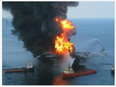
The burning Deepwater Horizon oilrig after an explosion caused by a design failure in the blowout preventer
