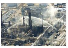
Emergency response workers fight secondary fires caused by the isomerization unit explosion at the Texas City refinery
