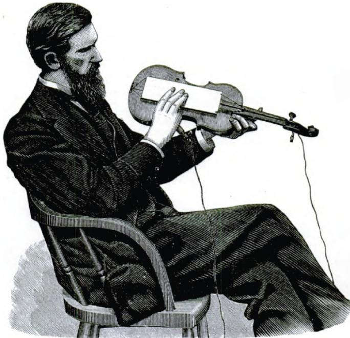
Figure 2.2. One of the first demonstrations of an audio-tactile display using electroadhesion (1874). Public domain image reproduced from [1].
