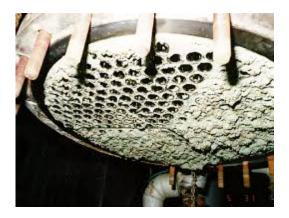
Figure 2: Fouled heat exchanger (regonline.com)
