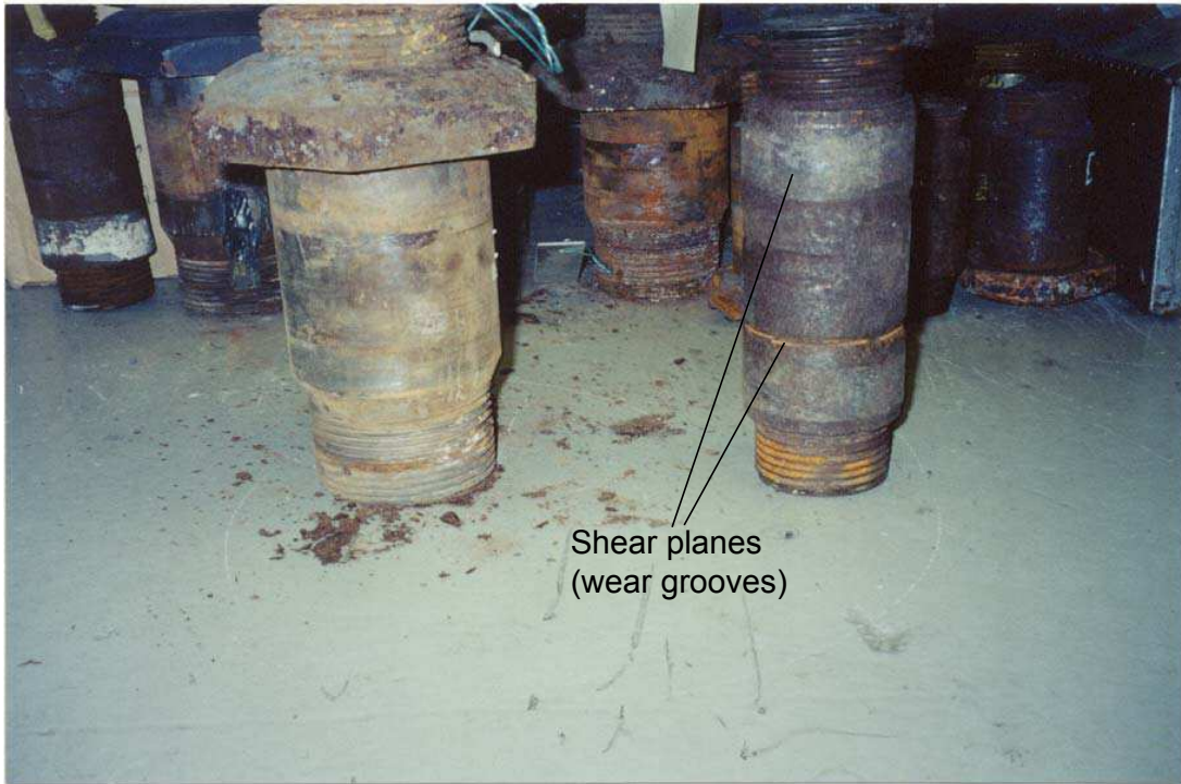
Figure 2.7. Shallow defects or wear grooves (Removed pins)
