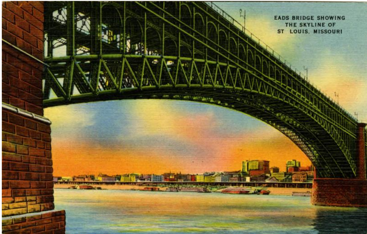
Figure 8: Eads Bridge (RT66260, Newberry Library)
