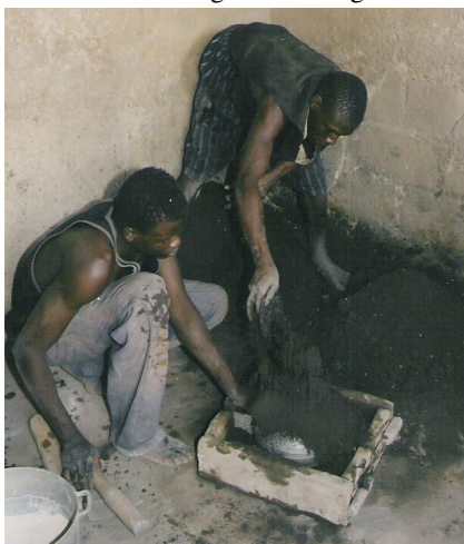
Photo 16. Filling the frame with sand ( tando ).
