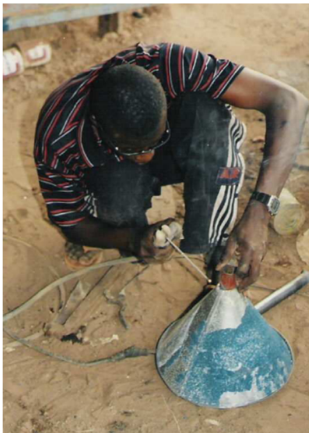
Photo 61. At the welder's shop, welding the tube at the bottom of the funnel.
