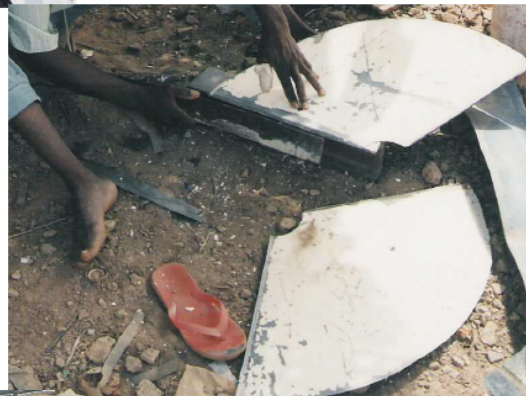
Photo 52. Knocking the edge to make a lip, in order to form a U-shaped channel.
