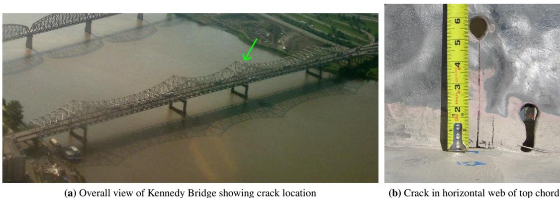
(a) Overall view of Kennedy Bridge showing crack location
