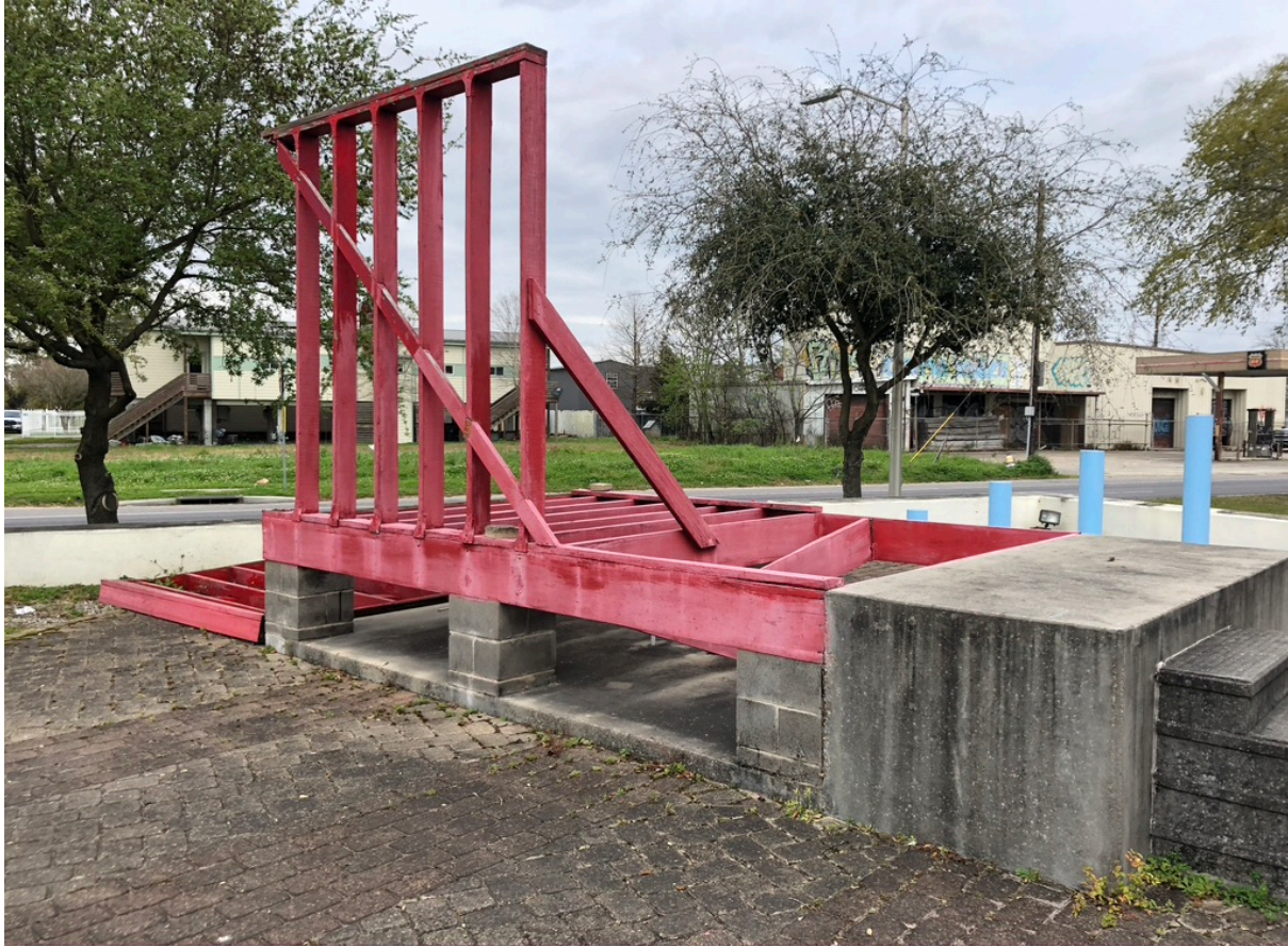
Figure 16. The Hurricanes Katrina and Rita Memorial in full. Note the collapsed wall behind the structure, the blue pillars at right, and the missing beams (and partially visible collapsed beam) directly behind the front concrete slab. Photo by the author.
